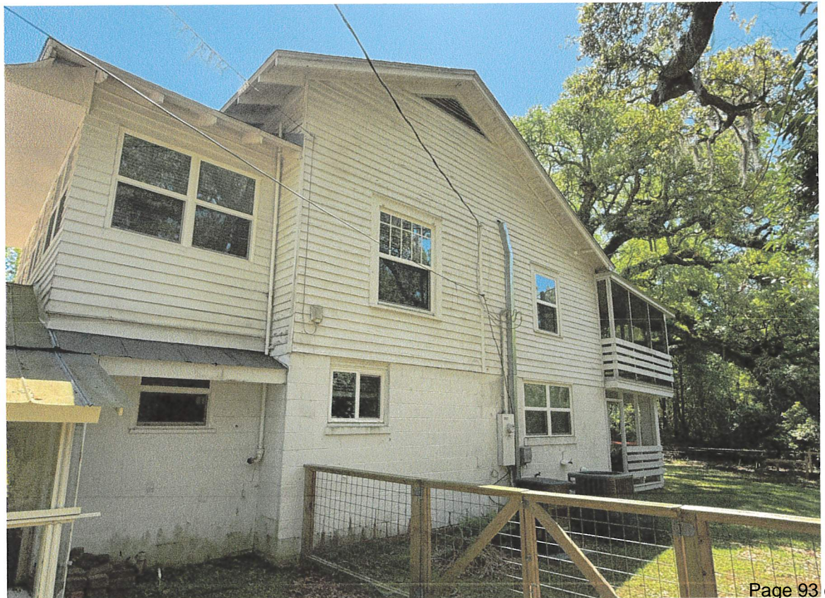
West side of home
