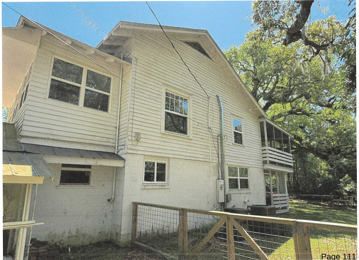
West side of home
