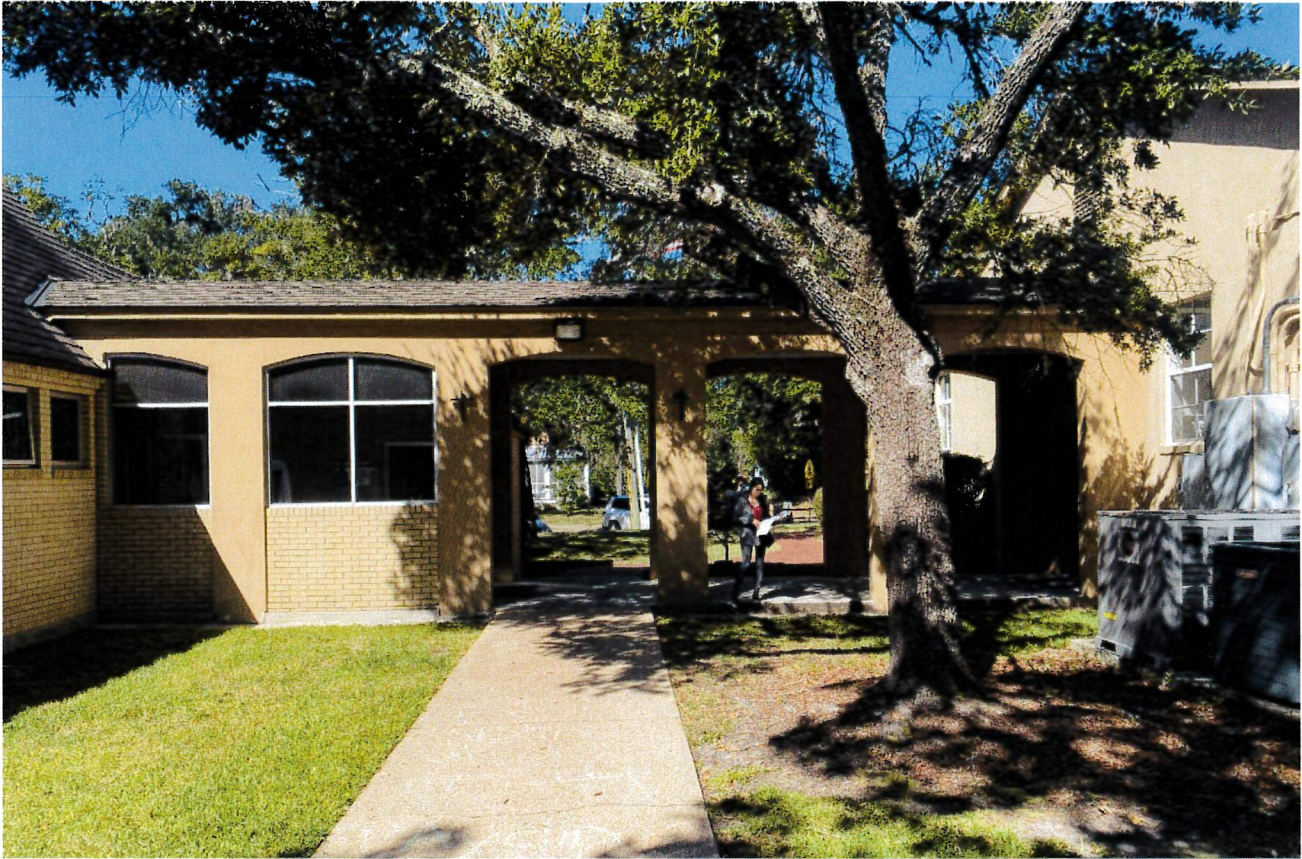
View of Church to School Connector from the East
