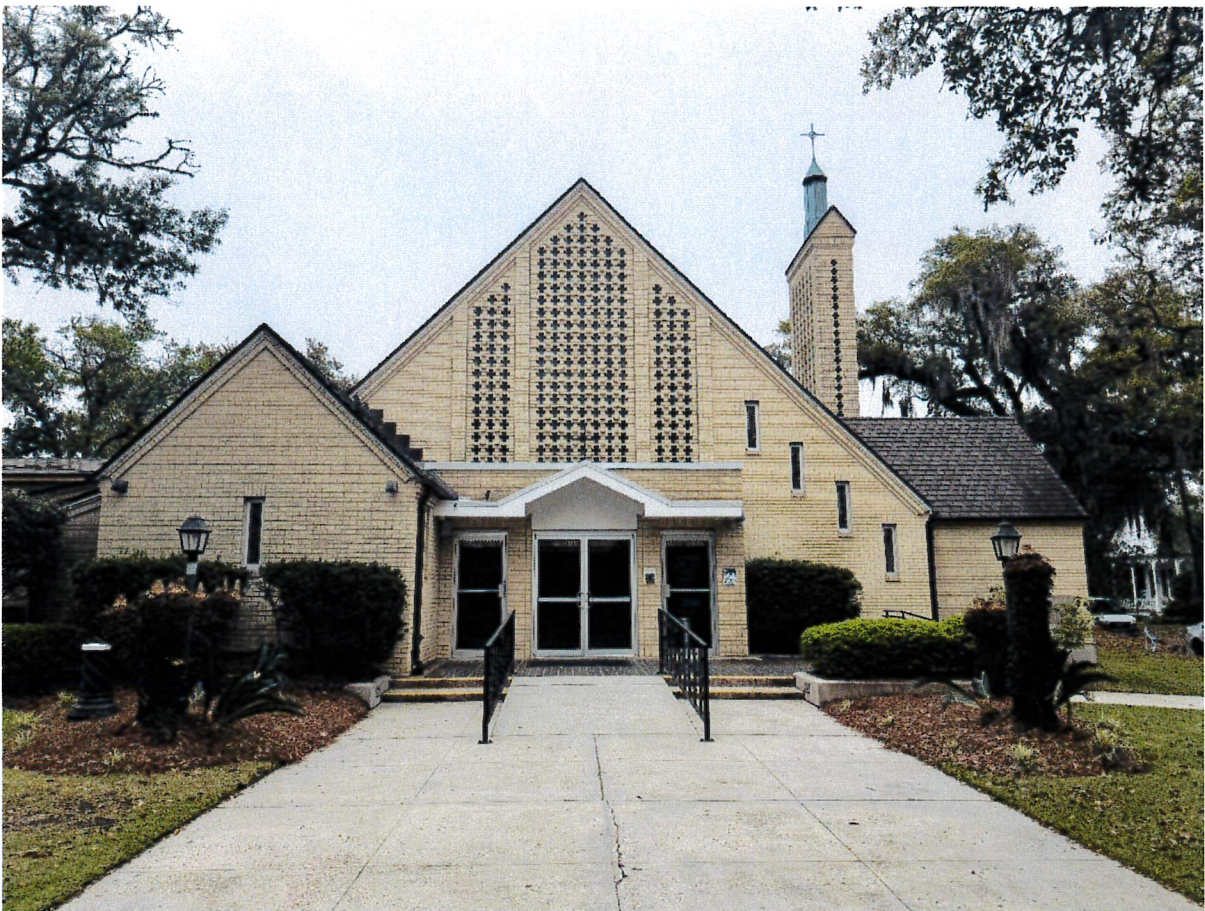
View of front of Church from Jackson Street (West)
