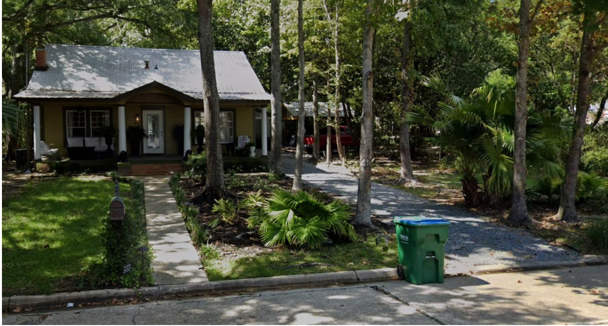
Figure 2. Existing Driveway and Walkway
