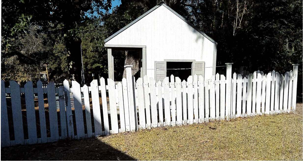
Figure 2. Existing 4' tall white wood picket fence
