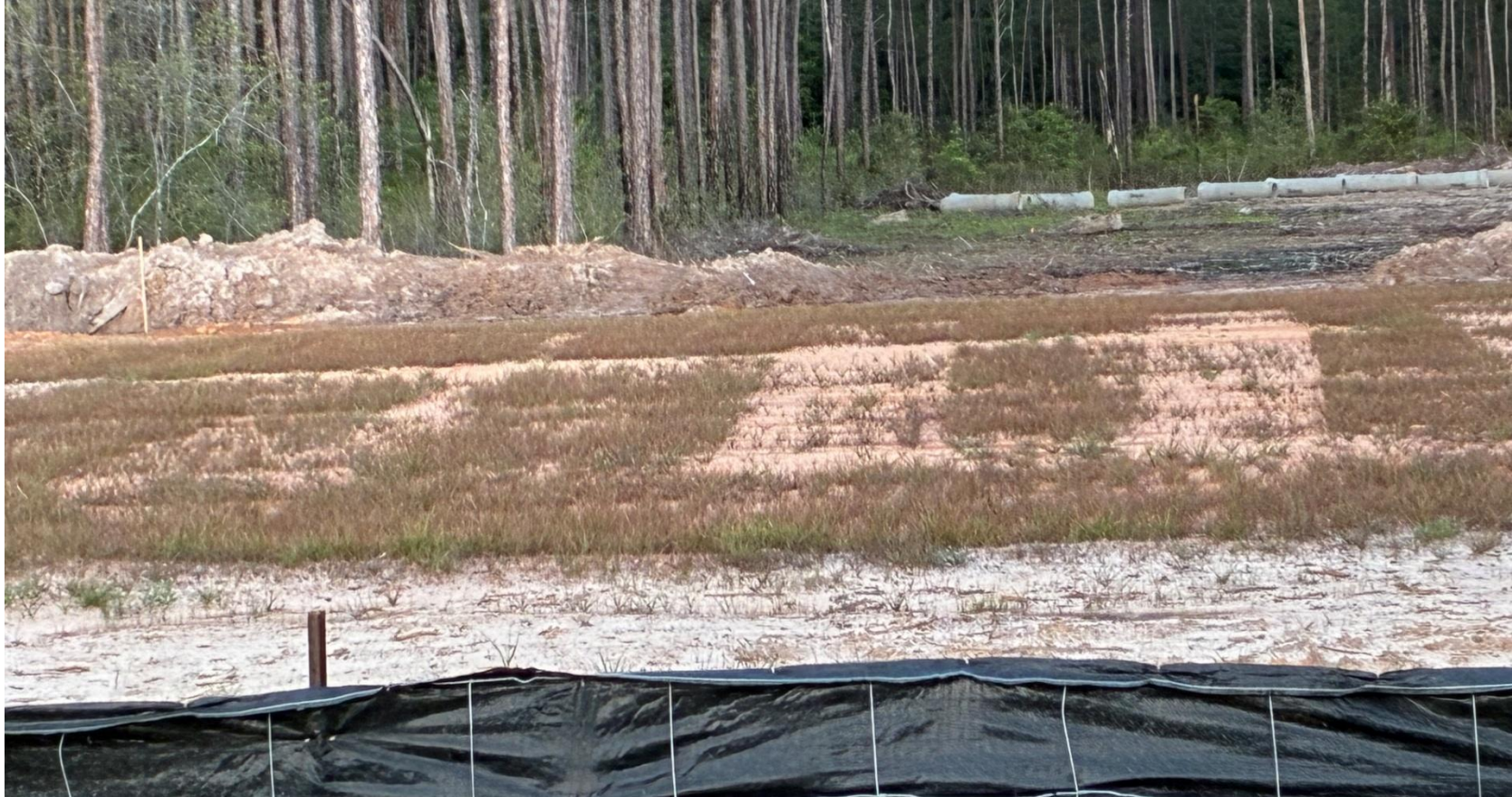
Photo 7: Looking east from Gibson Road, behind proposed lots 40-52; there is no erosion control between the current grading and forested wetlands/conservation easement
