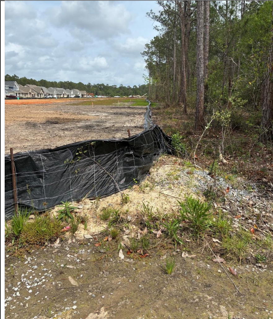
Photo 5: Looking east from the Madison Place 1 25' ingress and egress and drainage easement. This photo depicts 1-clearing into the proposed restrictive covenants I area and 2-single versus double silt fence; non-adherence to Condition 3 of the Storm Water Pollution Prevention Notes on the approved preliminary plat.
