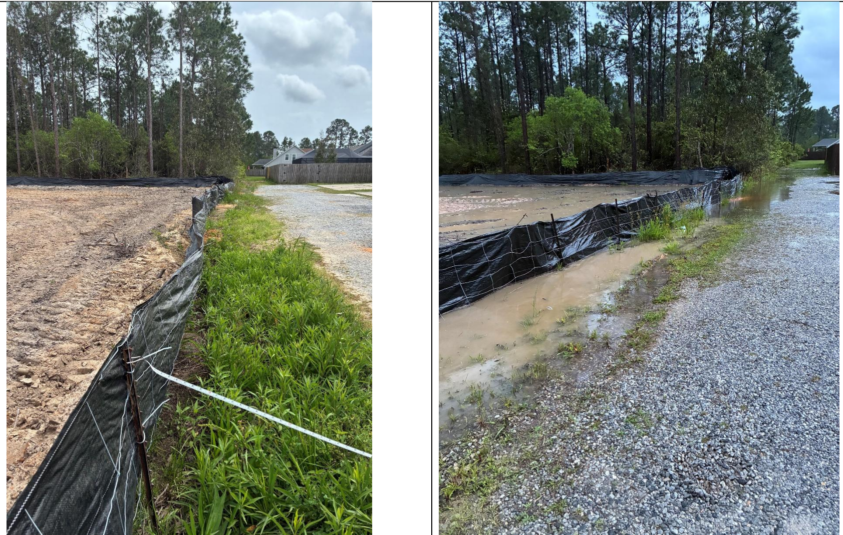
Photo 3&4: Looking South along silt fence (left photo); Looking south along silt fence. The silt fence is essentially in the centerline of the drainage ditch. This does not adhere to/violates Storm Water Pollution Prevention Notes 1, 3, and technically 6. Just after a rain event photo on the right depicting ineffective pollution prevention/sediment load in the ditch.
