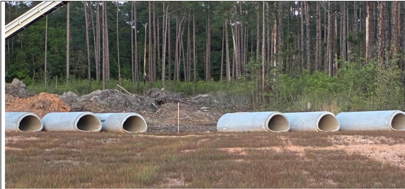
Photo 6: Looking east from Gibson Road, behind proposed lots 31-39; there is no erosion control between the current grading and forested wetlands/conservation easement
