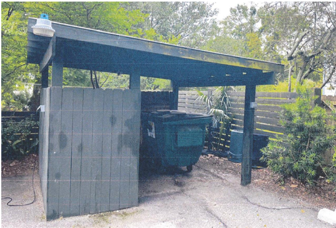
Figure 4: Current Dumpster Enclosure
