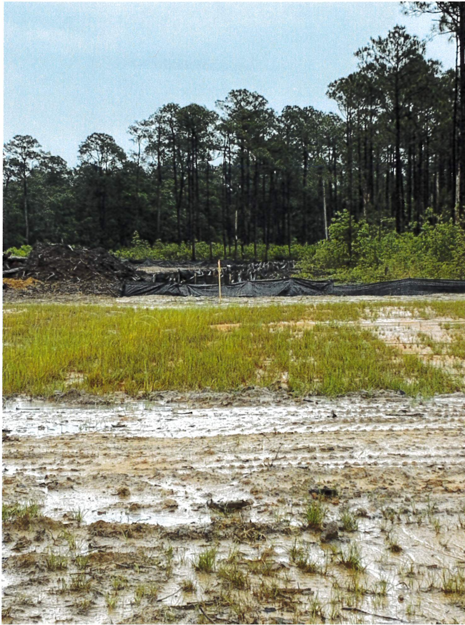
Photo 5: Looking east from Gibson Road, mechanized land clearing and topography alteration in the conservation easement behind proposed lots 31-39 in the conservation easement.
