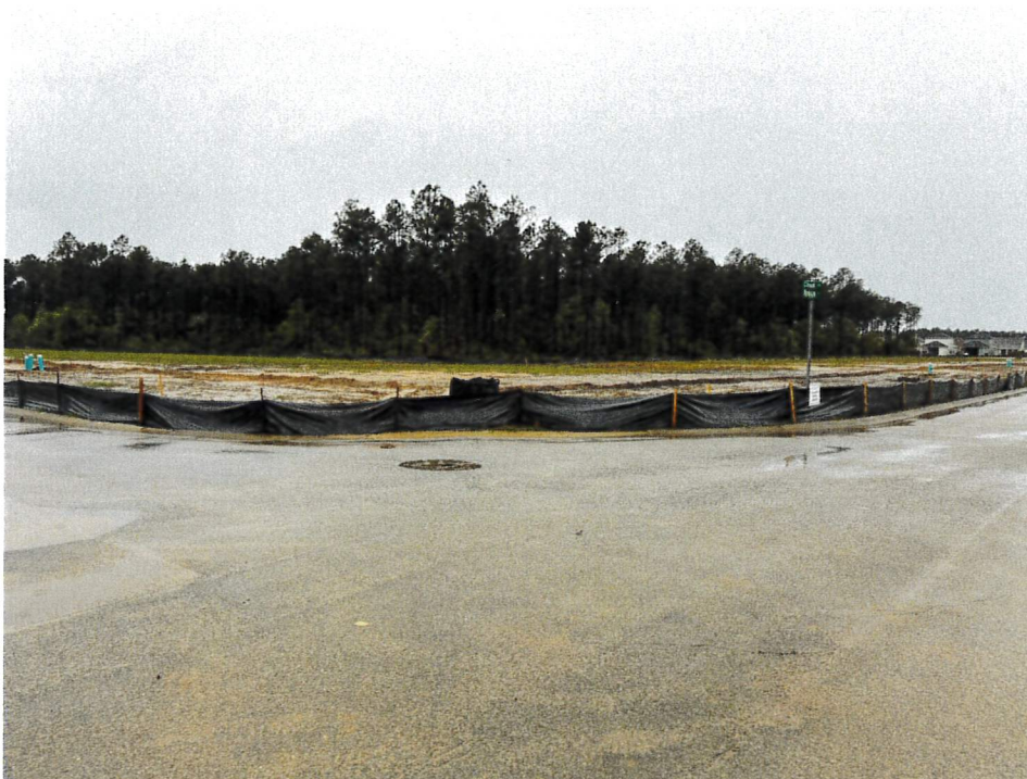
Photo 9: Mechanized land clearing and topographic alternation (filling) in the conservation easement at the corner of Madison and Gibson Road.
