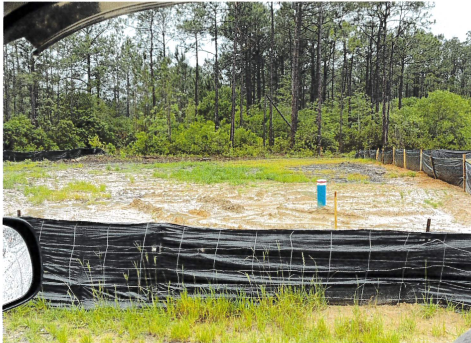
Photo 8: Mechanized land clearing and topographic alternation in the conservation easement south of Lot 21.
