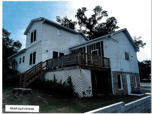
Figure 2,3,4,5. Existing Deck and Screened Porch
