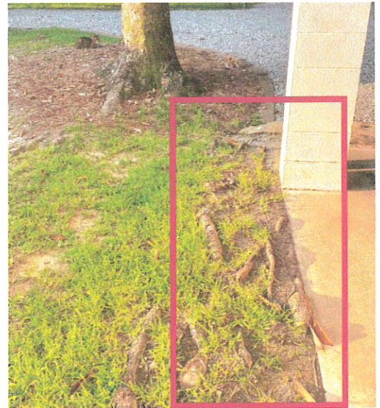
Foundation concerns and damage caused by roots
