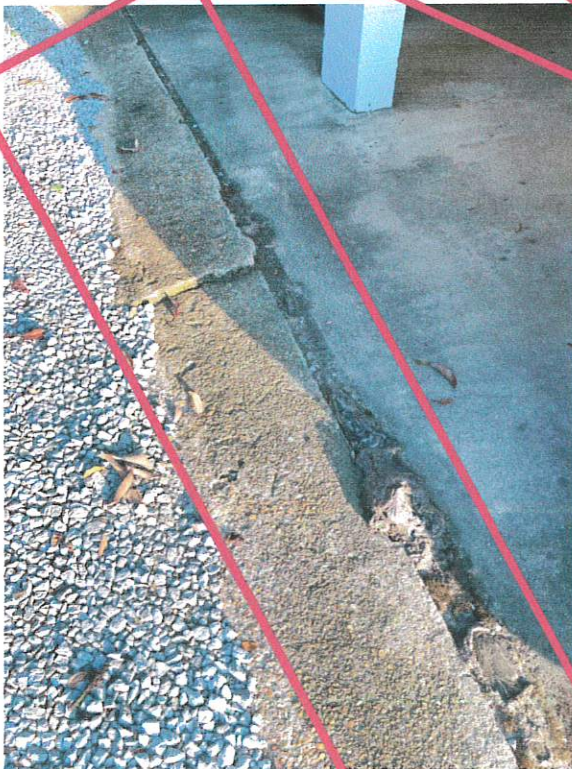
Foundation concerns and damage caused by roots
