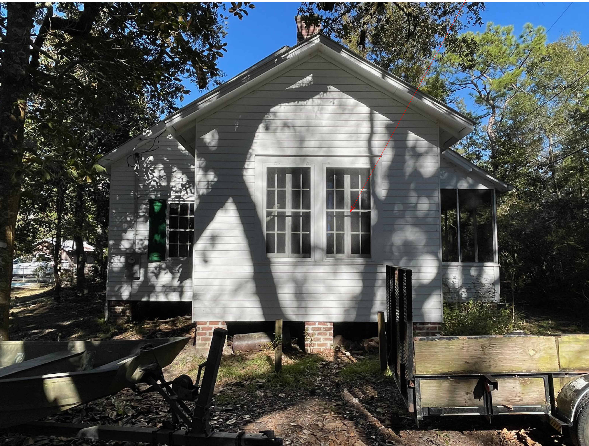
EXISTING ANDERSON HOME LOCATED ADJACENT TO PROJECT SITE
