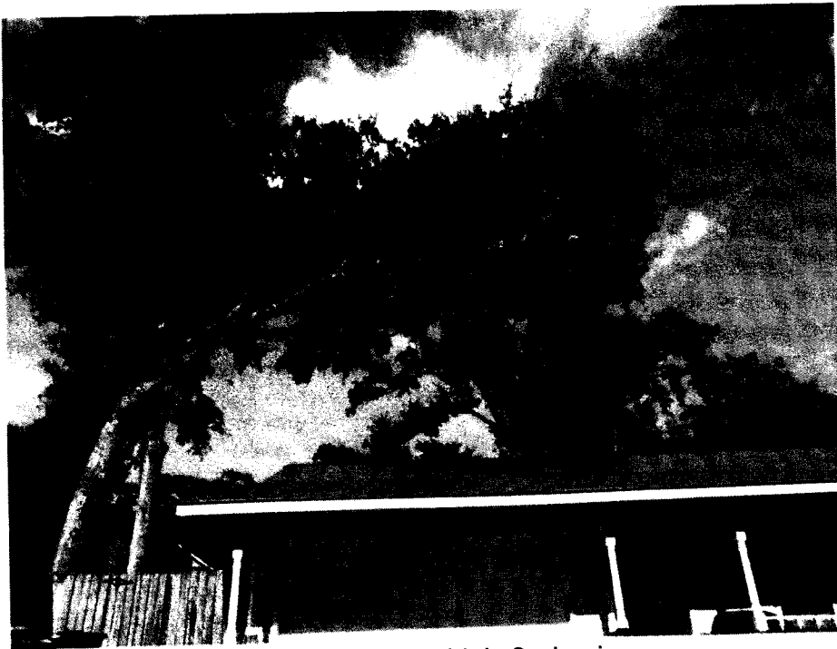
Premises Hazard - Trees/Limbs Overhanging
