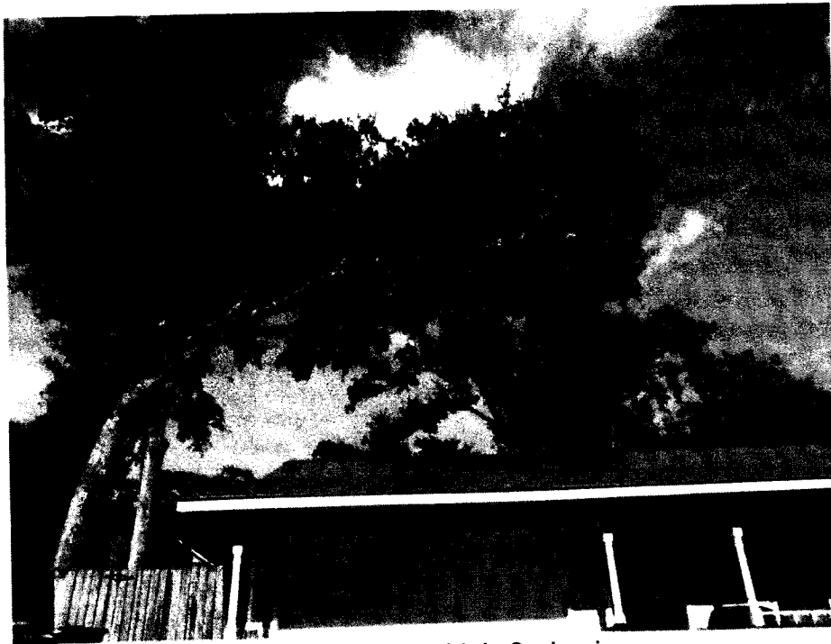
Premises Hazard - Trees/Limbs Overhanging
