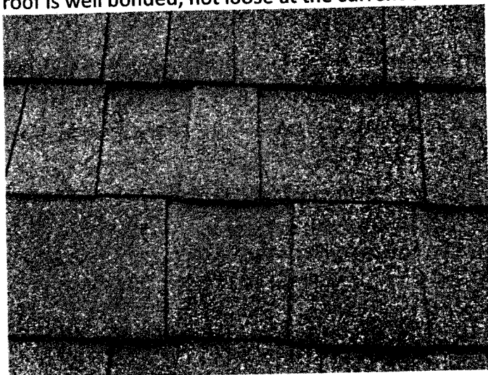
Example photo of roof cover
