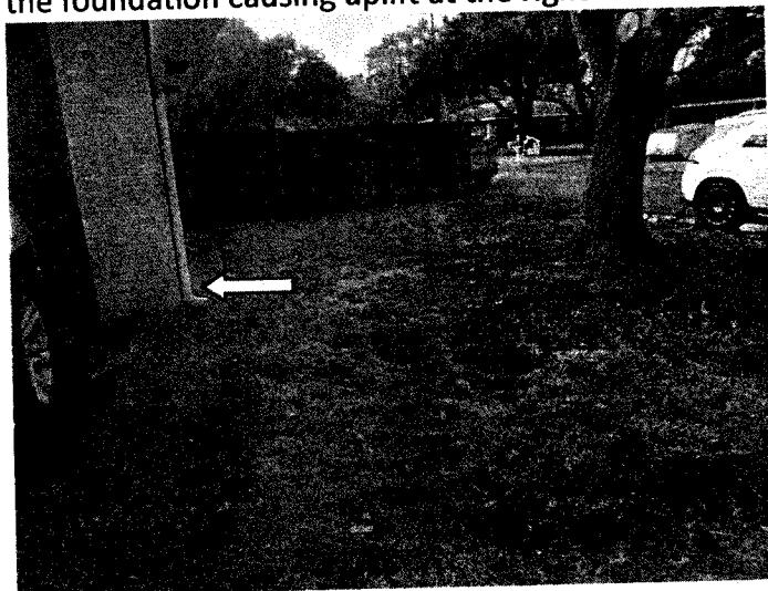
Tree at front right corner – roots encroaching Exterior Wall Hazards, Cracking, Continued
