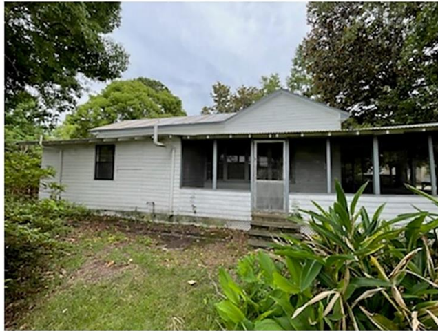
Left Side of house – Looking South
